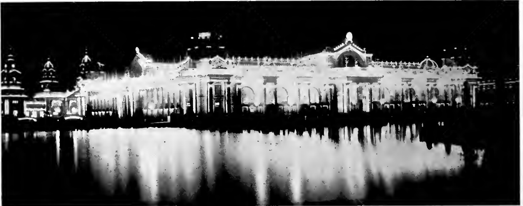
FIG. 20.—A VIEW OF ELECTRICITY BUILDING BY NIGHT.
